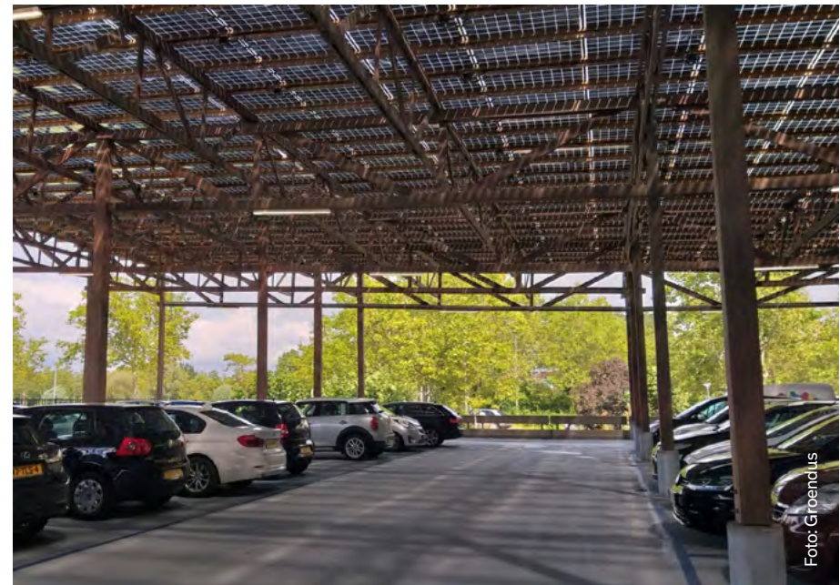
Solar carport in Heerlen
